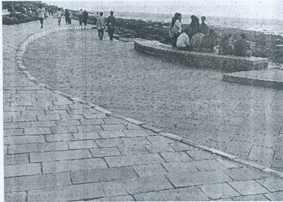
Bandra Bandstand after the redevelopment work
